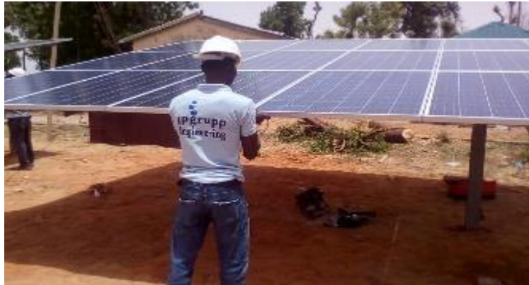
IPgrupp Technician Installing PV Panel on a Client Site
