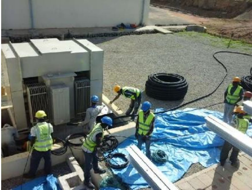
IPgrupp Engineers/Technicians complete installation Of 1MVA 11/0.4KV step-up transformer for Solar Plant Tie-in to Grid
