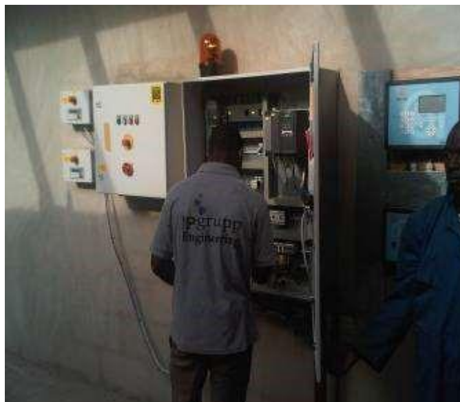
Commissioning an Automated feed and Egg collection Panel for a Client with Extensive Investments in state of the art agricultural equipment
